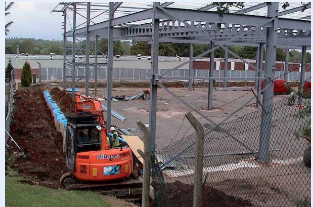
Stage 4: Make sure that the presence of the root barrier membrane is recorded and is not disrupted by future developments and landscaping.
